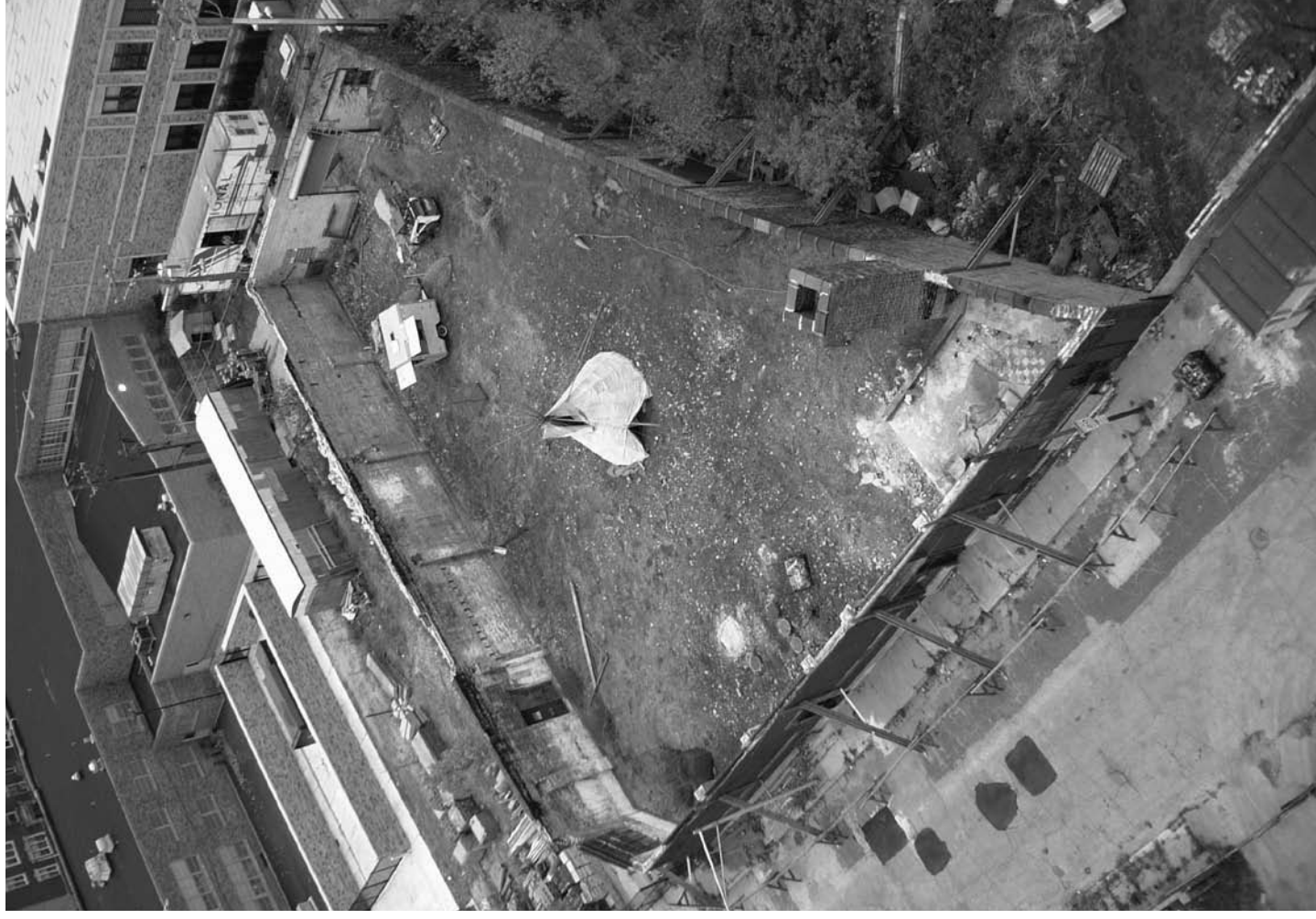
The Experimental Station after the removal of the fire damaged parts of the building, Chicago, photo Dan Peterman, 2001
